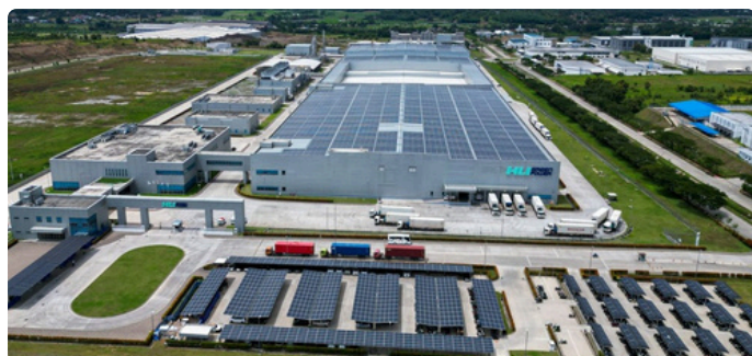
HIJAU completed the installation of a 7,144 kWp rooftop solar PV system at PT HLI Green Power's factory in Karawang in September 2025.
