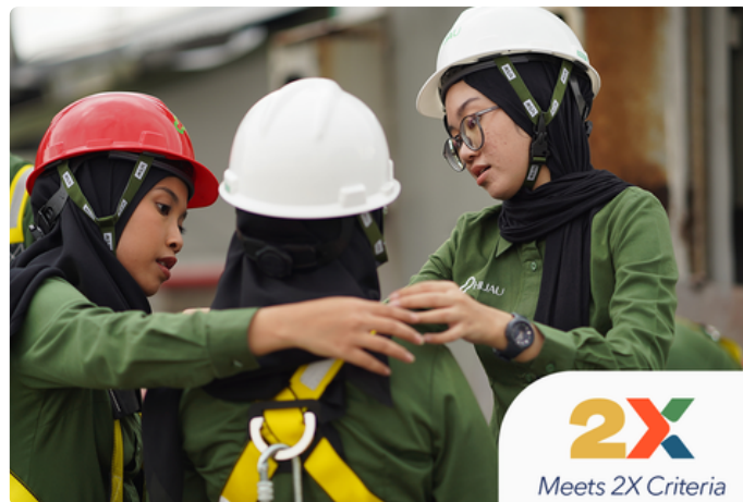
HIJAU's female engineers preparing for installation of solar PV system
