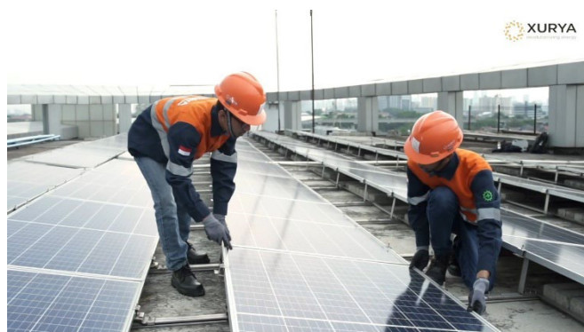
Xurya engineers performing maintenance work at a solar rooftop site
